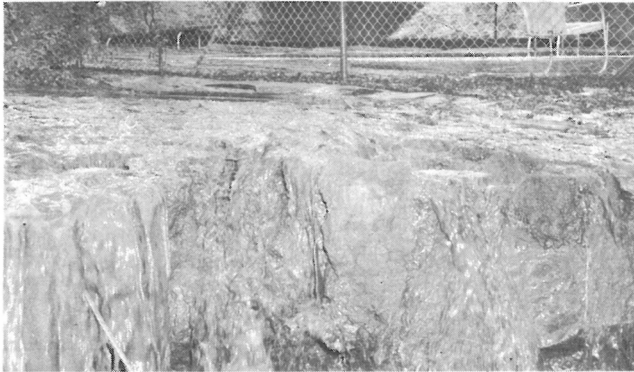
SMALL NIAGARA TORE OUT TONS OF EARTH AT HOLIDAY RANCH. THIS SHOWS TORRENT DROPPING SOME FOUR FEET OVER EDGE AS IT CUT AWAY EARTH, WASHED IT AWAY.
